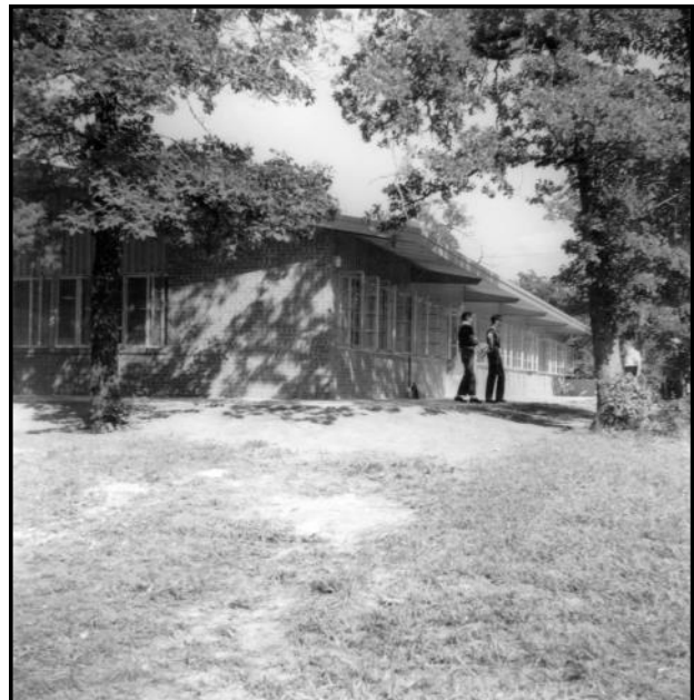
1962 North West side of Dinning Hall.
